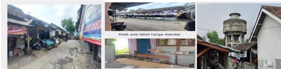
Figure 5a. The condition of Kranggan Market is that there is no parking space, no price tags for the goods sold, no cleaning/sanitation facilities, and the water tower is no longer functioning.
