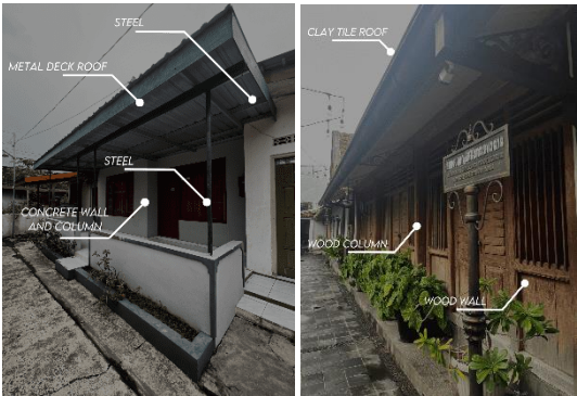
Figure 11. The materials used in RW 09 are still traditional, such as wood and clay, while in RW 07, they have been modernized to concrete and steel. (Source: Author’s Documentation, 2024)
