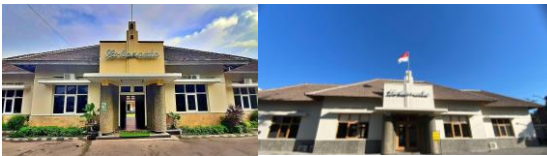
Figure 11. Lokananta’s Facade in 1956 and 2023 (Source: https://surakarta.go.id/ and Author Documentation, 2023)
