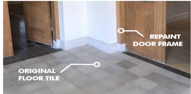
Figure 19. Architectural Element Maintain and Changes at Museum Lokananta (Source: Author Documentation, 2023)
