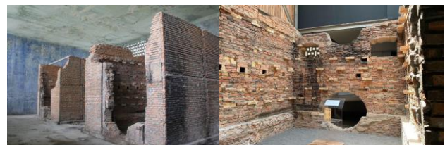
Figure 10. Boiler Room Before and After Revitalized (Source: facebook.com/rumahatsiri and Author Documentation, 2023)
