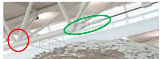
Figure 2. The joint construction of the KJT roof uses a combination of welded and pin.
