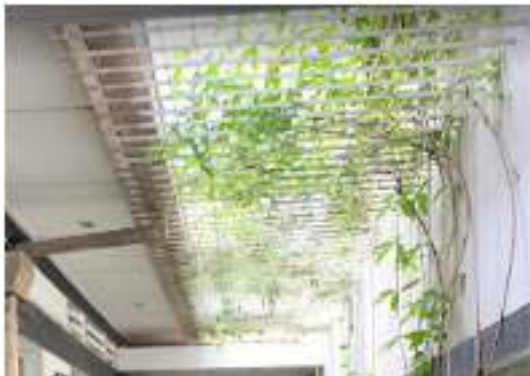
Gambar 10. Skylight Surabaya C2O Library and Collabtive (sumber: Dokumen Penulis, 2023)
