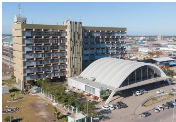
Figure 1. Beira Station (Source: Chaves et al., 2022)
