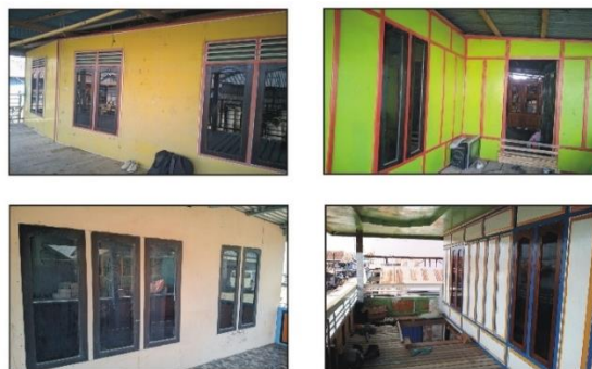
Figure 4. Condition of Openings in the Walls of the Bajo Tribe's Stilt Houses (Source: Author's Document, 2026)
