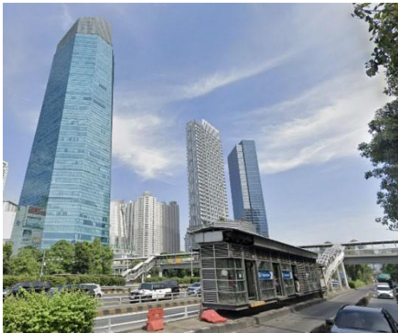
Figure 2. Tanjung Duren Halte (East) and Pedestrian Overpass with Existing Buildings (Source: Google Maps, 2025)
