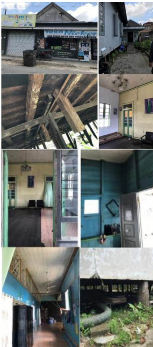
Figure 5 Condition of house C
