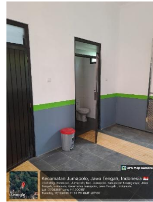
Figure 11. Toilet of Mandiri Putra Karanganyar Special School
