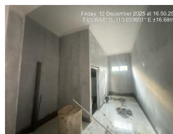
Figure 17. Toilet of Mutiara Bangsa Kendal Special School (Source: Mutiara Bangsa Kendal Special School's Document, 2025)
