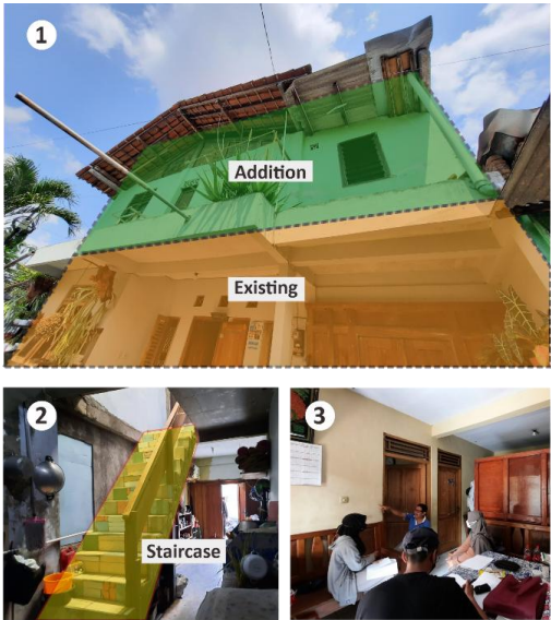
Figure 4. (1) Vertical addition above the existing mass in case 2; (2) Proper staircase connecting the first and second floors; (3) Interior space constructed with appropriate dimensions and materials (Source: Author's Document, 2025)
