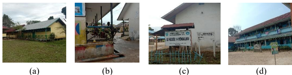
Figure 1: Post flood school (a) at state elementary school Sungai Ringin (a), at state elementary school Sungai Kawat (b), at state elementary school Mengkurai (c), and at state elementary school Sintang.
