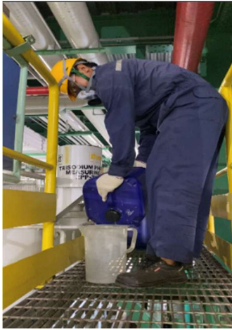
Figure 3. The Process of Neutral Amine Filling Manually
