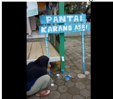
Figure 2. Installation of Directional Signs for Karang Asri Beach
