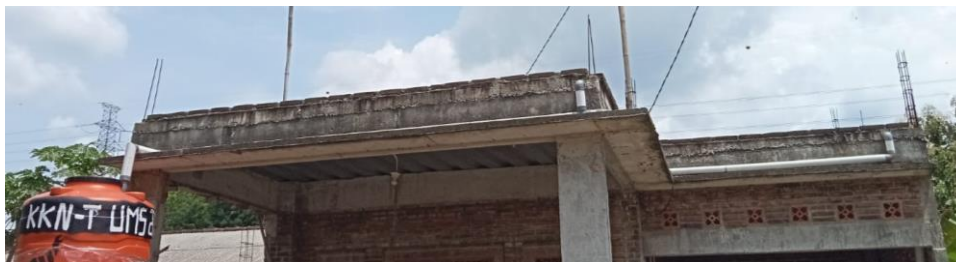
Figure 2. Water Line Pipe
