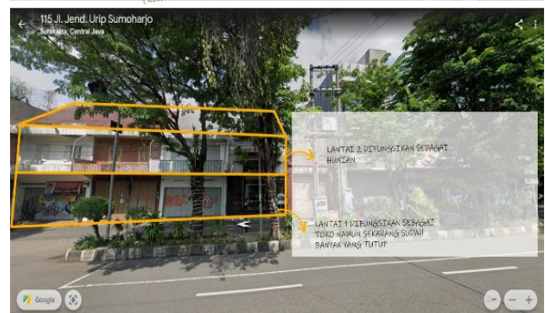
Figure 6. Existing Segment B-C Condition (Source: Author Document, 2024)
