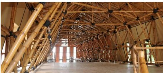
**Gambar 10.** Modular sambungan bambu MPP (Madan Puraskar Pustakalaya) (Sumber : <https://abari.earth/mpp>, diakses pada 18 November 2023)
