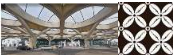
Figure 4. The roof at the drop-off area in YIA airport with batik kawung configuration.
