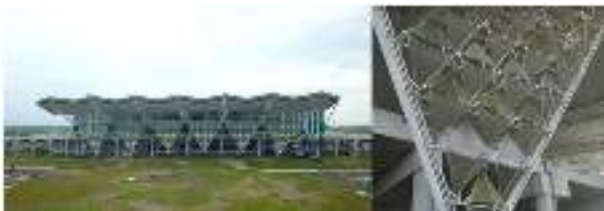
Figure 3. Perforated metal shade in the drop-off area of KJT airport.
