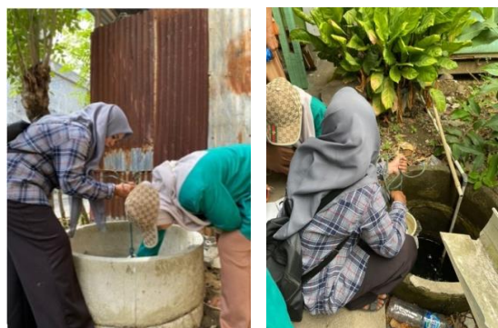
Figure 6. The location of the Phreatic Well is Outside the Residents' Houses.
