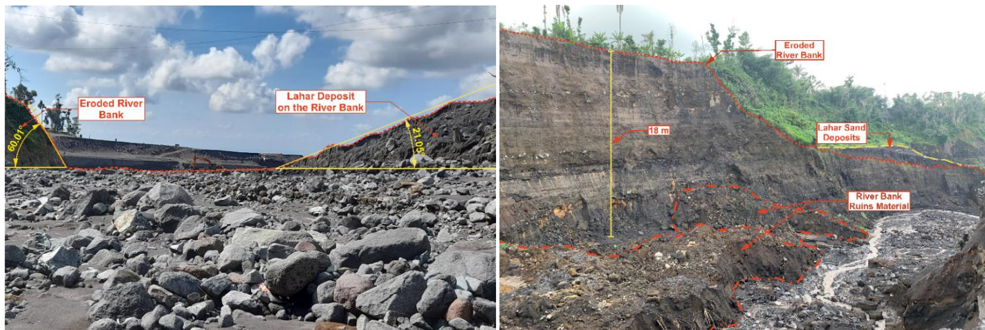
Figure 6. Changes in river cliff morphology due to being covered by lahar material (right), remnants of river cliff collapse by lahars with large frequency and energy (left).
