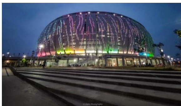
Figure 11. Lighting System on the JIS Façade (Source: Author Documentation, 2024)
